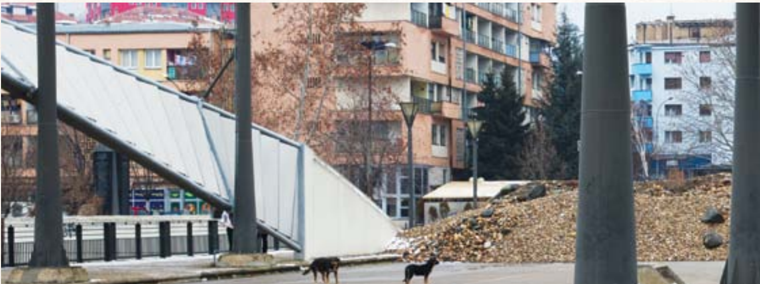
The bridge across the Ibar river, both connecting and dividing the city of Mitrovica in Kosovo, remains a symbol for ethnic divisions in the Balkans.
