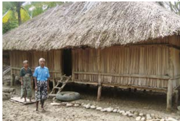
Raising the houses is a protection from flooding. Although local construction materials are used, they are still too expensive for the poorer villagers
