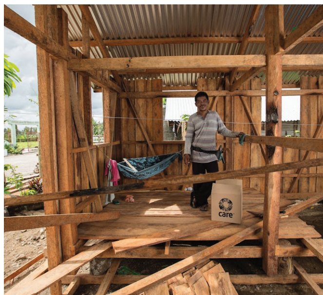
CARE helped families rebuild their homes following Typhoon Haiyan in the Philippines. ©Tom Platzer/CARE
